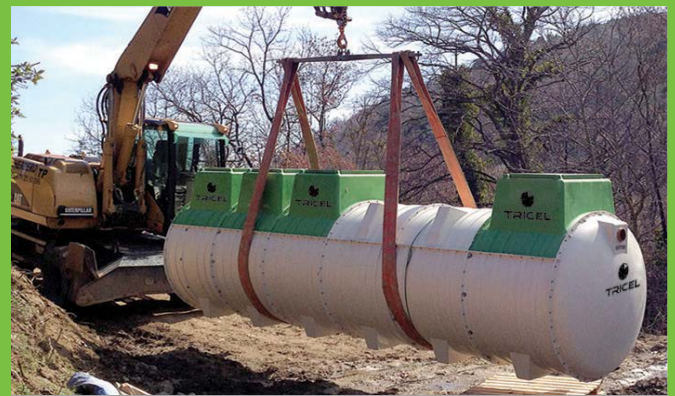
Installation of Tricel Novo FR20
